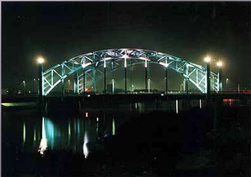
Meiwa Bridge, Edogawa-Ku, Tokyo
